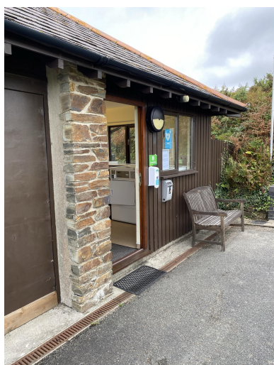
Entrance into Laundry and Information Room
