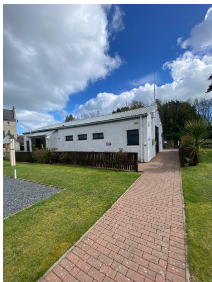
Main Toilet Block
