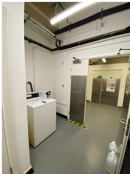
Dishwashing and Washing Machine Room
