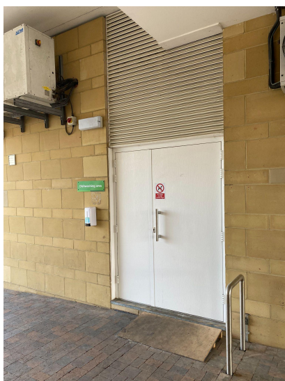
Door to Dishwashing and Laundry Facilities
